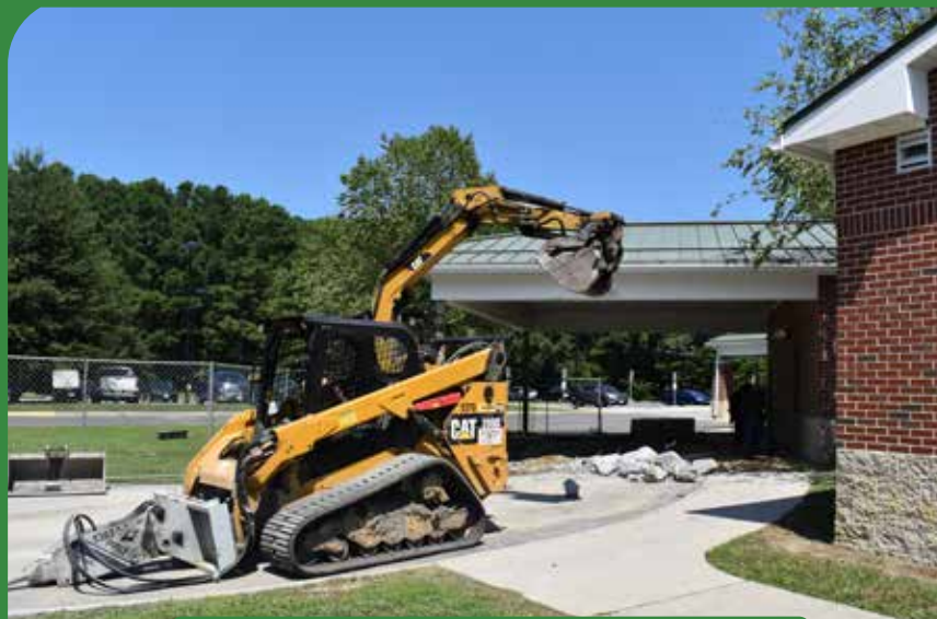
Onley Community Pharmacy ground breaking.
